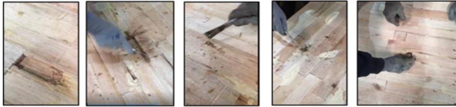
Figure 1. Picture of product defect
